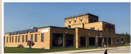
Reed River Trading Company Building open for business.
